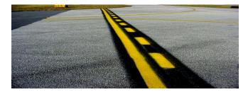
Instrument landing system (ILS) hold lines (ILS holding position markings) are painted onto the surface at locations where it is necessary to keep aircraft and vehicles on the ground from interfering with the signals transmitted from the ILS antennas. When ILS approaches are in progress, during periods of low-visibility, operators may be instructed by ATCT to "hold short of the ILS critical area".
