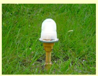
Designed to identify the edge of the usable runway surface at night and during periods of low visibility.
